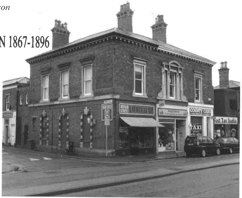
Building on the corner of High Street and Monson Street, Lincoln.
